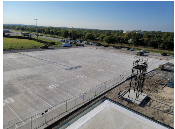
Site: Band striping and tower relocation complete.
