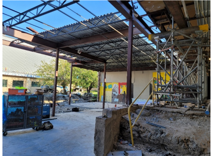
Area T: Structural steel installation in progress.
