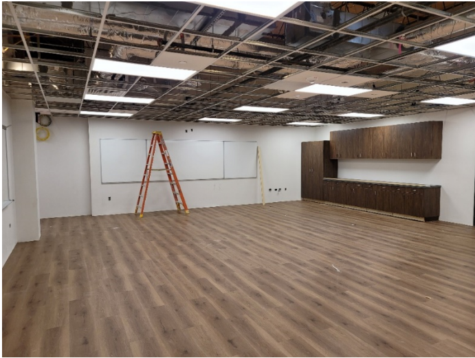
Area N: Casework installation in progress.
