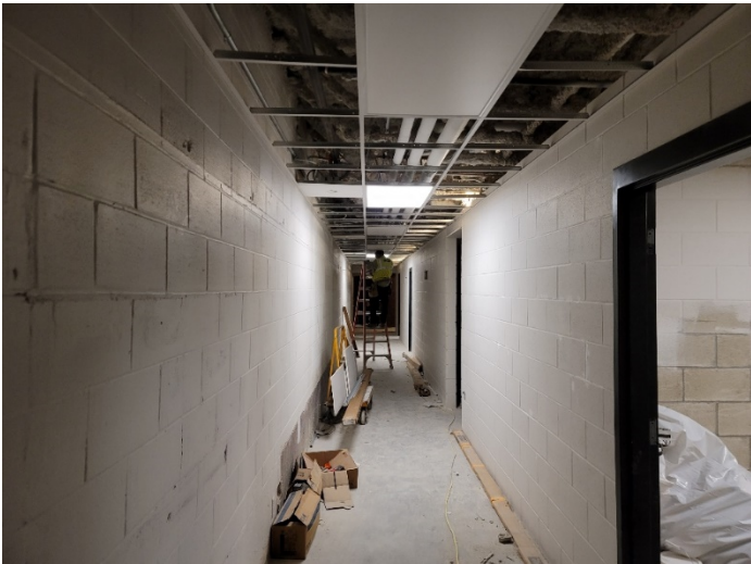
Area D: Ceiling framing and MEPT ceiling trimout in progress.
