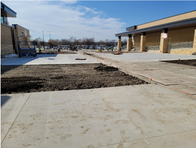
Area D&T Courtyard: Topsoil installation in progress.
