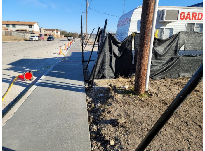
Site: Installation of fencing along Atkinson in progress.
