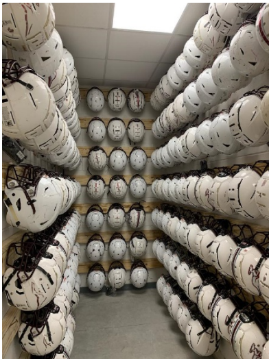
Area P: Wood blocking for helmets complete.
