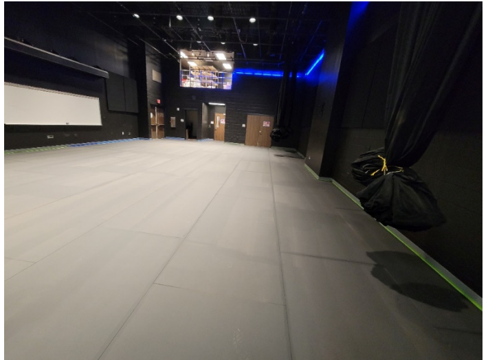
Area K: Black Box Flooring Complete.
