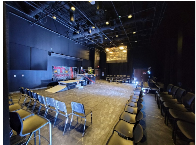
Area K: Black Box Flooring Complete.
