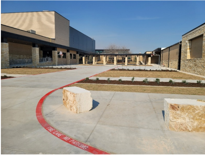
Area D&T Courtyard: Landscaping, striping, and basketball goal installation complete.
