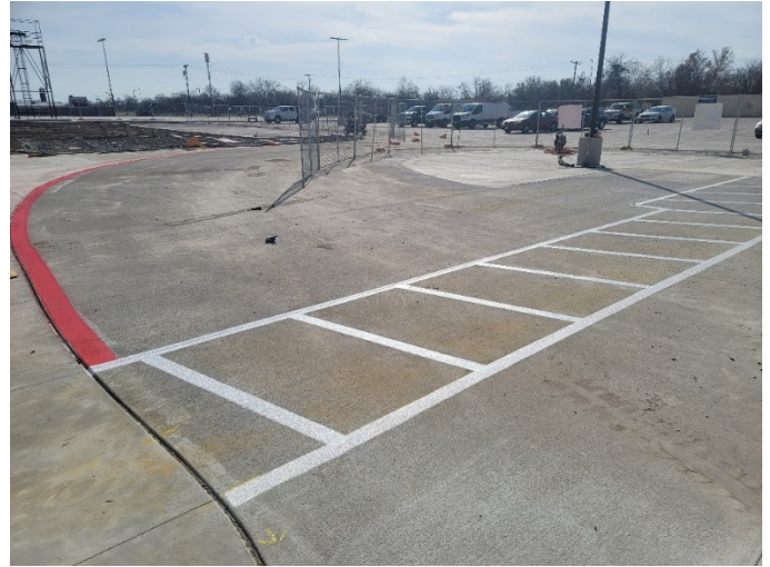
Area D&T Courtyard: Striping in progress.
