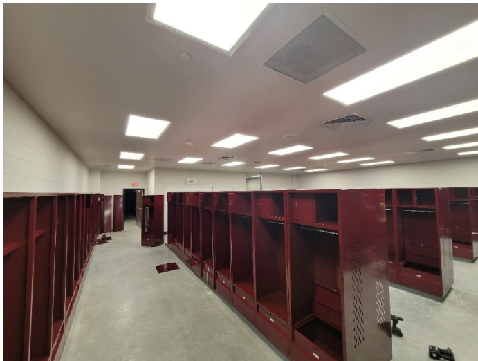
Area P: Locker installation in progress.
