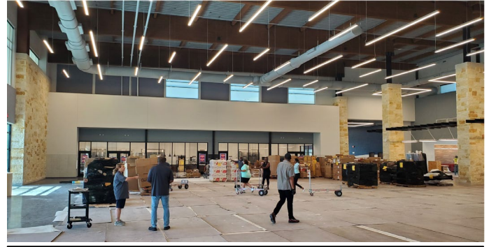
Building: KISD stocking continues in Area G for distribution into the building.
