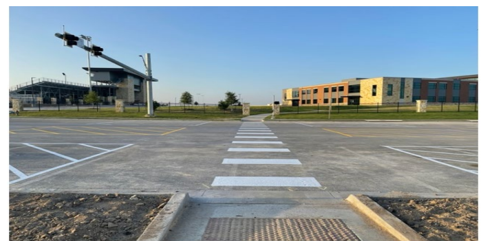
Site: Chaparral Road striping in progress.
