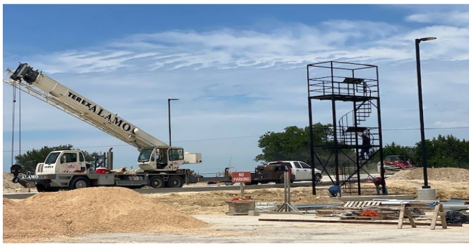
Site: Band Tower installation is in progress.
