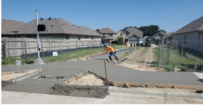
Site: Sidewalk being placed and finished for access in neighborhood.
