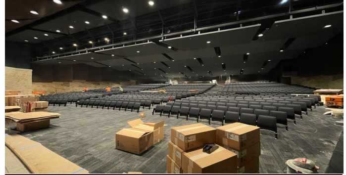
Building: Auditorium seating installation in progress.
