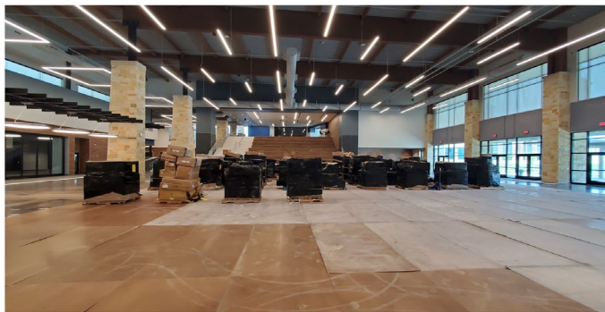
Building: KISD stocking in progress in area G.
