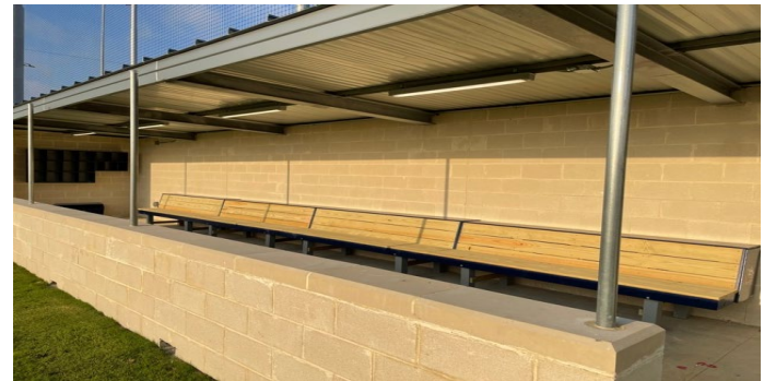
Site: Baseball and softball benches and helmet storage installation is complete.
