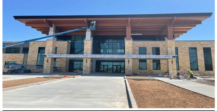
Building: Soffit panel installation nearing completion at front entrance.
