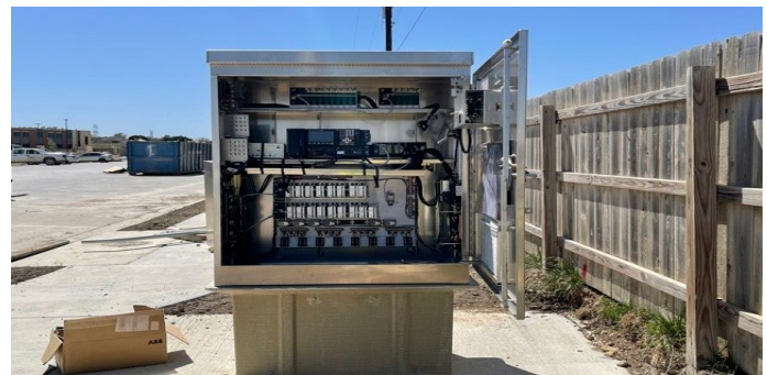
Site: Pedestrian Beacon System installation in progress.
