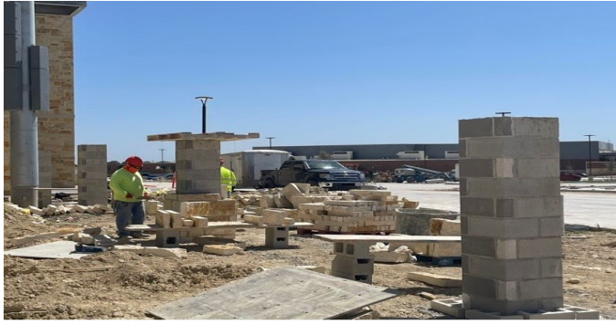
Site: Masonry columns near Pressbox being built.
