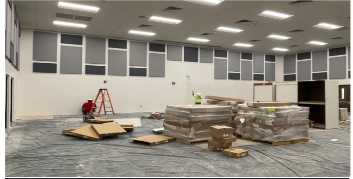
Building: Paint in progress in Fine Arts area.
