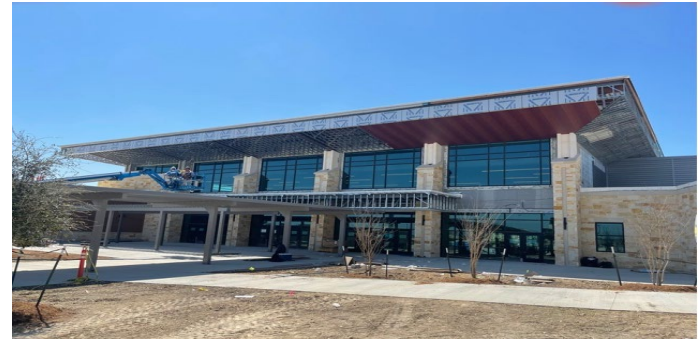
Building: Area G east entrance soffit panel installation in progress.
