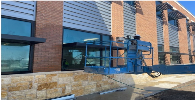
Building: Water testing in progress.
