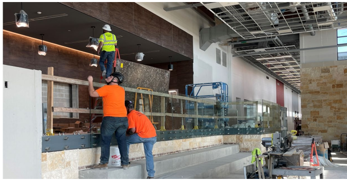
Building: Glass rail installation in progress at auditorium lobby.
