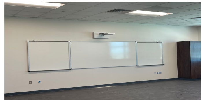
Building: Projector arm installation in progress in Area E classrooms.
