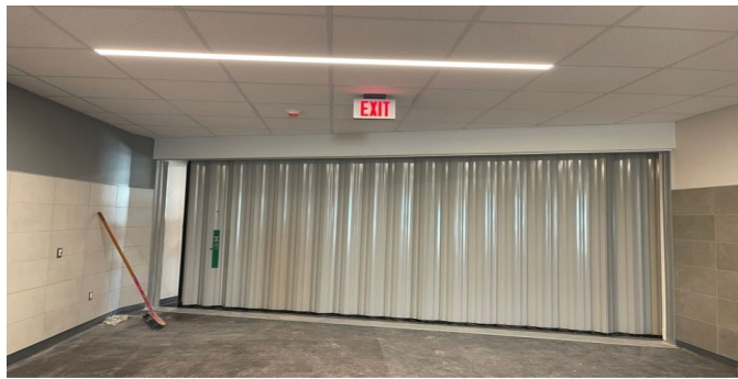
Building: Accordion fire door installation in progress.
