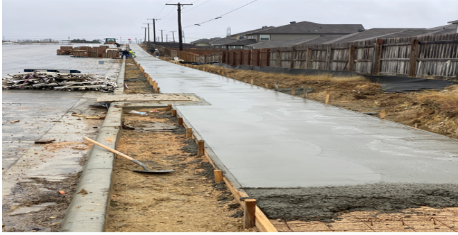
Site: City sidewalk along Chaparral Road in progress.
