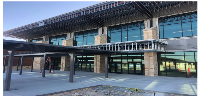
Building: Concrete flatwork completed at east entrance to Commons.
