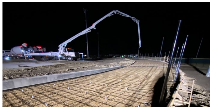
Site: Sidewalk being placed and finished near baseball field.
