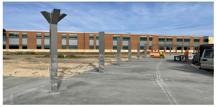
Site: Canopy installation in progress on east side of buildings.
