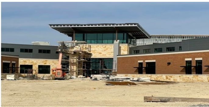
Site: South side column masonry in progress.
