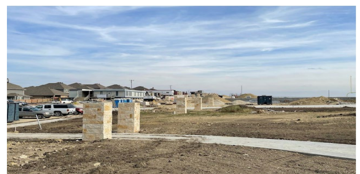
Site: Site masonry columns installation continues.
