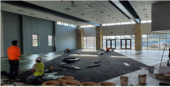
Building: Area G Media Center carpet installation in progress.
