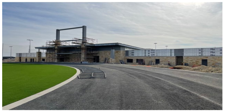
Site: Football Concession masonry in progress on video display board columns.
