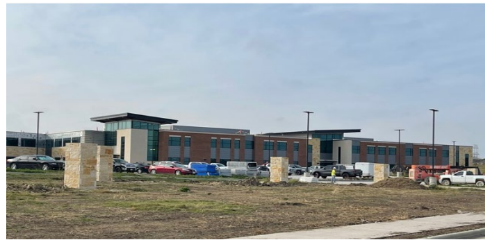
Site: Site masonry columns in progress along Chaparral Road.
