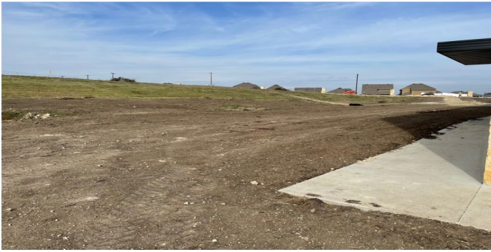
Site: Topsoil being spread around building perimeter.
