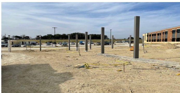
Site: Installation of canopy footings at teacher's parking lot.
