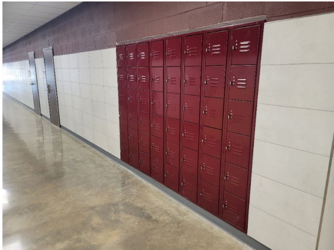
Area P: Laundry locker installation in progress.
