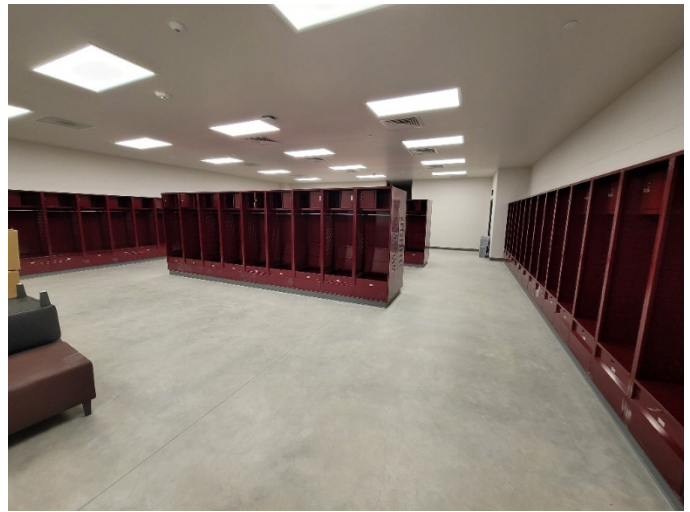
Area P: Varsity football locker installation in progress.
