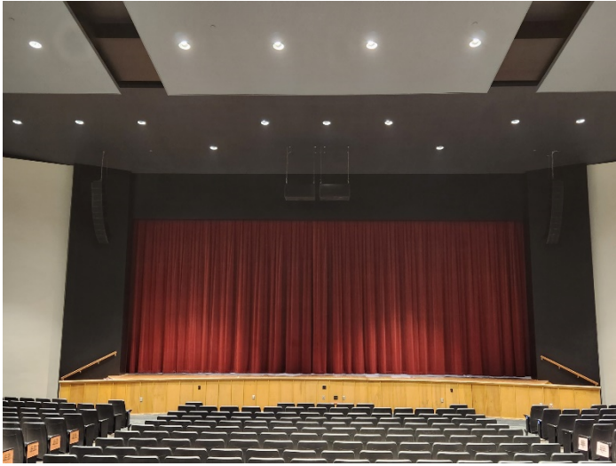
Auditorium: Speaker and lighting installation complete.
