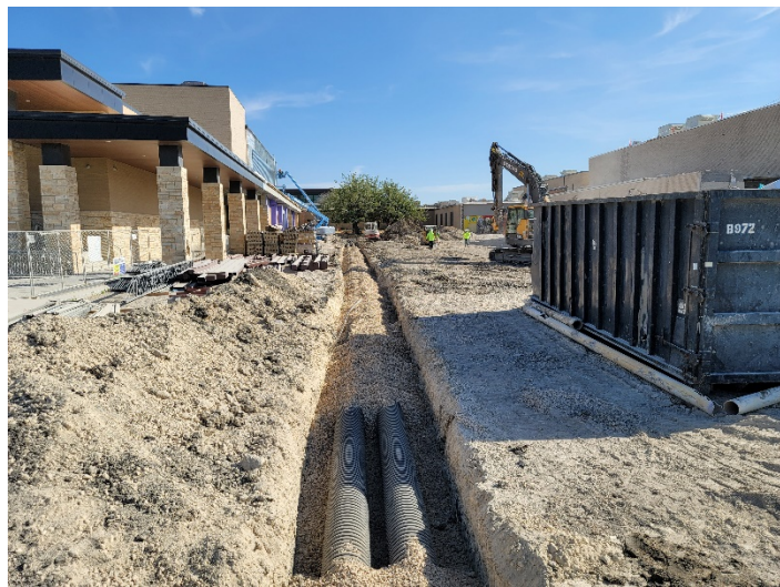
Area D&T Courtyard: Underground utility installation in progress.
