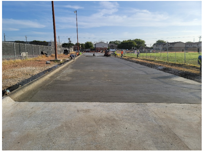
Site: Paving installation in progress.
