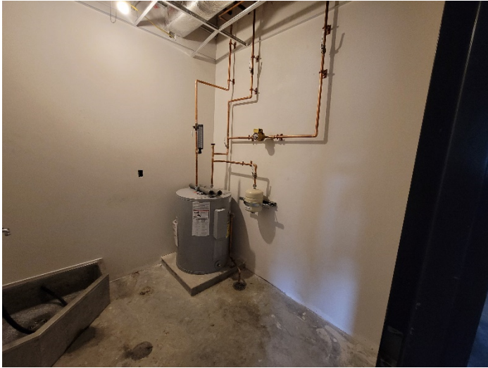
Area M: Water heater installation in progress.
