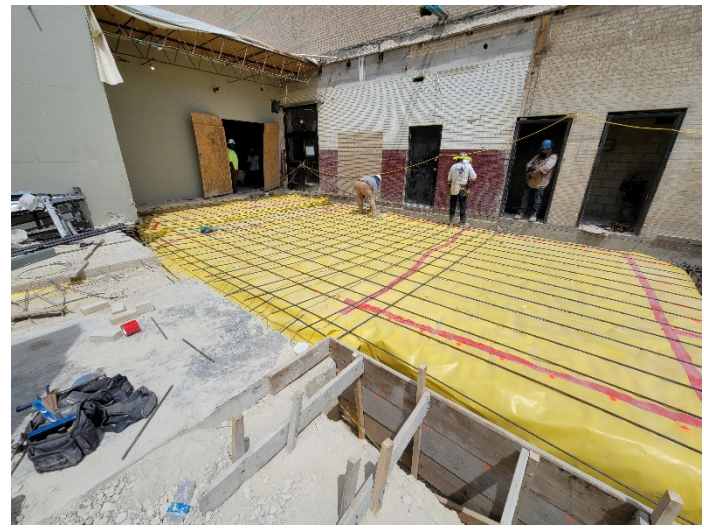
Area D: Foundation reinforcement installation in progress.
