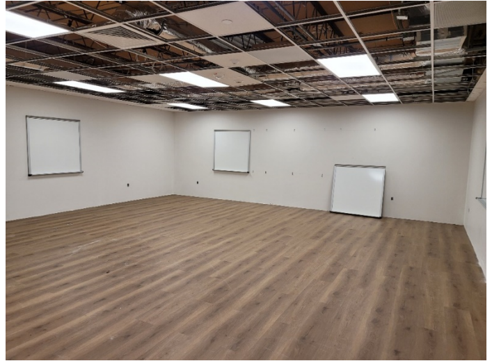
Area M: MB & TB installation in progress.
