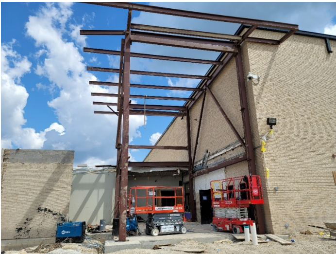
Area D: Structural steel installation in progress.
