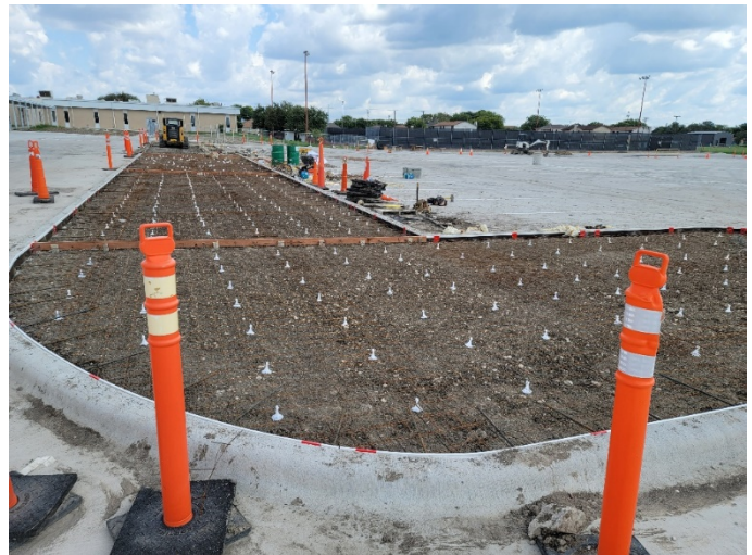
Site: Sidewalk and flatwork installation in progress.
