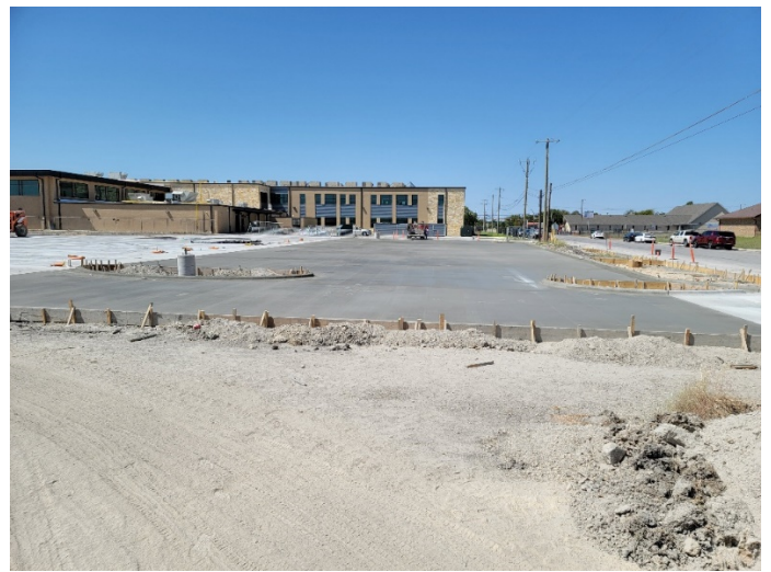
Area M&N Parking: Paving installation in progress.
