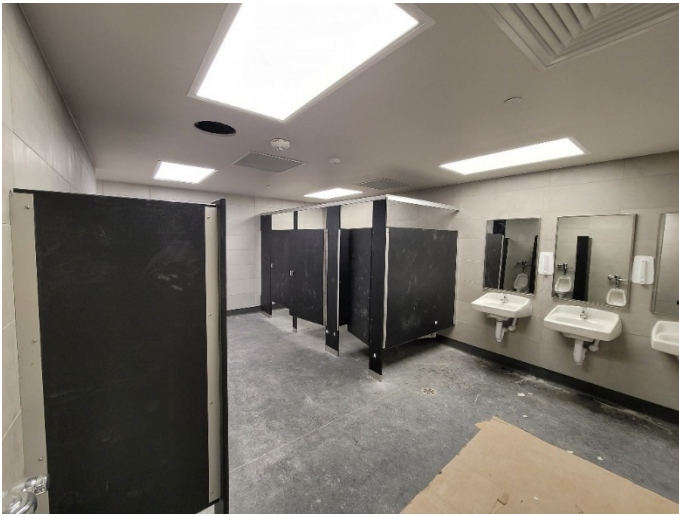
Area M: Toilet partition and accessories installation complete.
