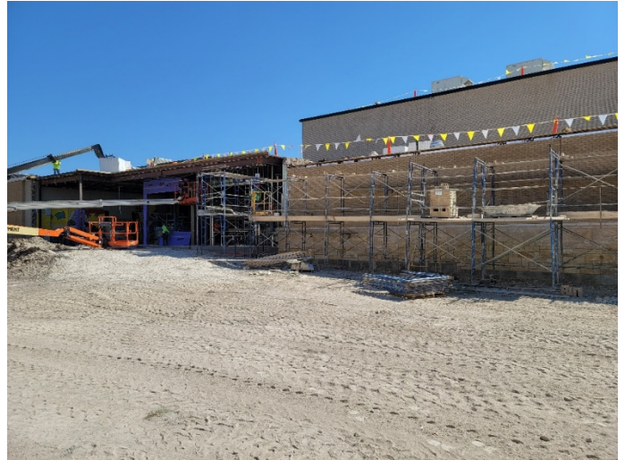
Area D&T: Exterior masonry and framing installation in progress.
