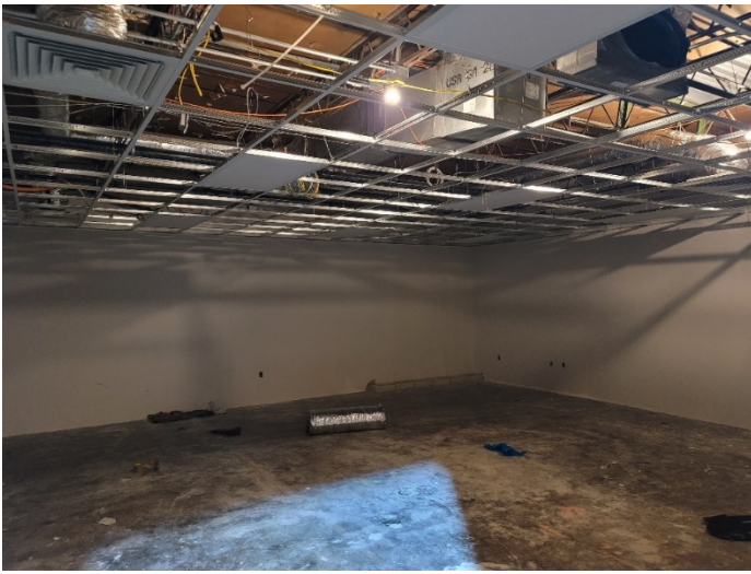
Area M: Ceiling grid installation complete. MEPT ceiling trimout in progress.
