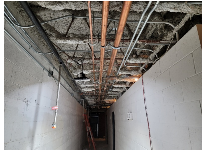
Area D: Overhead MEPT rough-in in progress.
