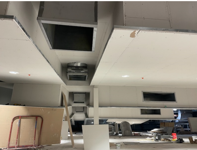
Auditorium: Sheetrock installation in progress.
