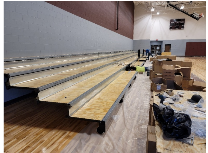
Area L: Bleacher installation in progress.
