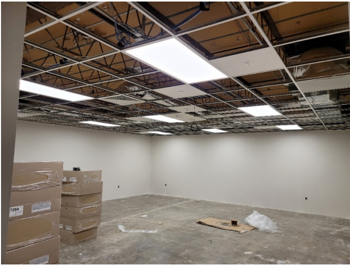
Area M: Lighting installation in progress.
