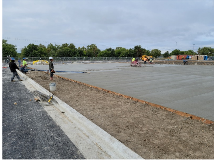
Site: Band practice field installation in progress.
