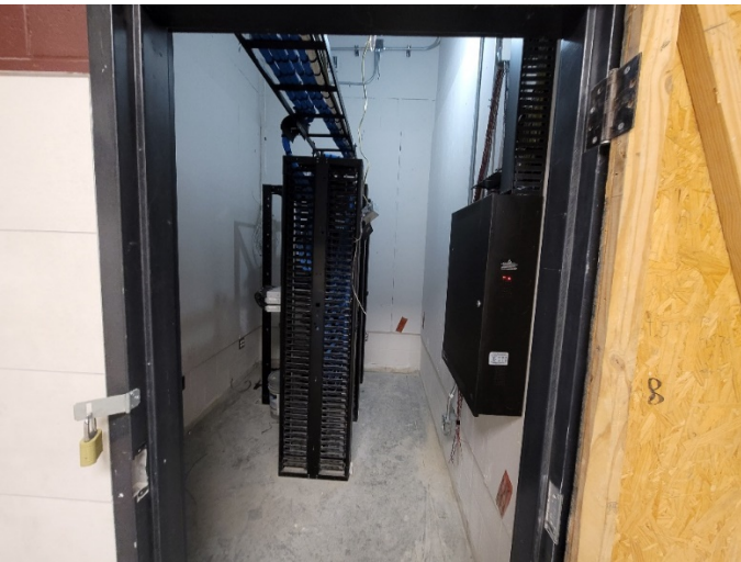
Area P: IDF closet build-out in progress.
