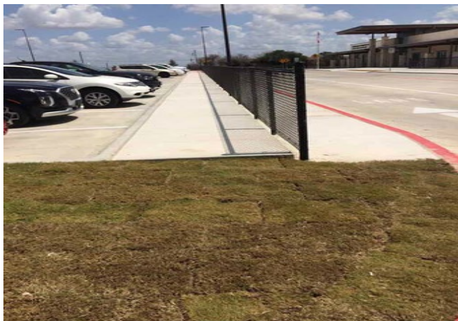
Interior: Final fencing at paving is completed.
