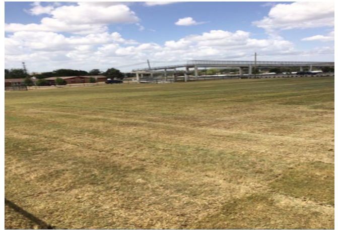
Exterior: Sod has been installed in front field.
