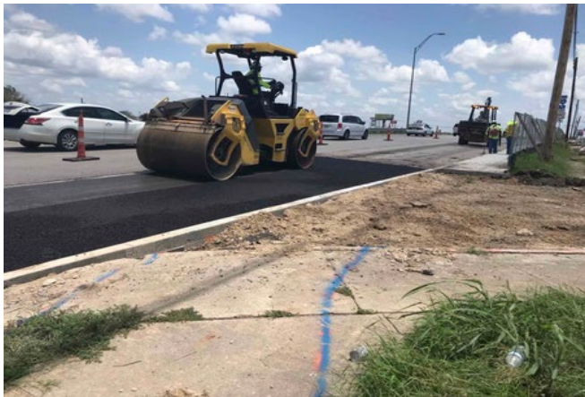
Exterior: Rebuilt curb at access road with new asphalt.
