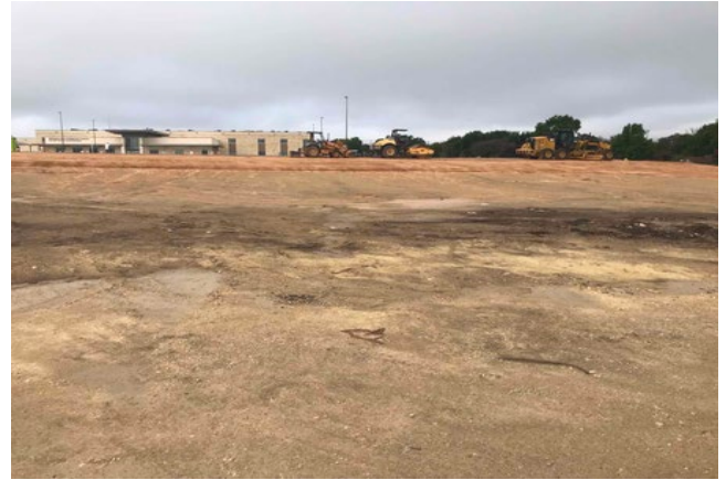
Exterior: Final grading around new parking lot
