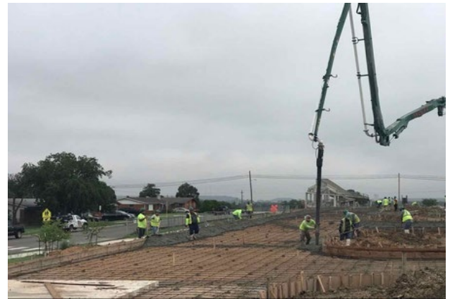
Exterior: Final concrete pour for new drive.
