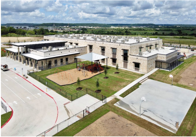
Exterior: Sod and landscaping installed. Hydromulch down and watered.
