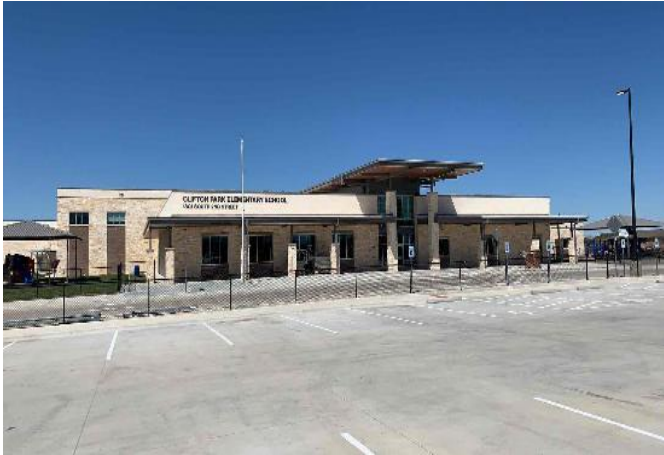
Certificate of Occupancy received.
