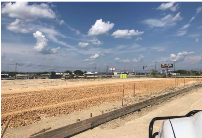
Exterior: Forms for concrete are going in.
