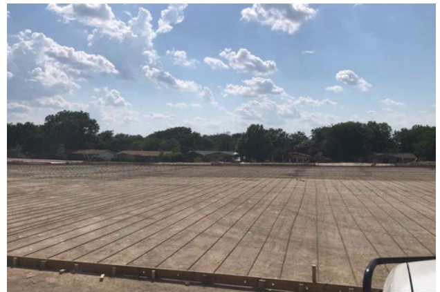
Exterior: Forms and rebar for concrete are going in.
