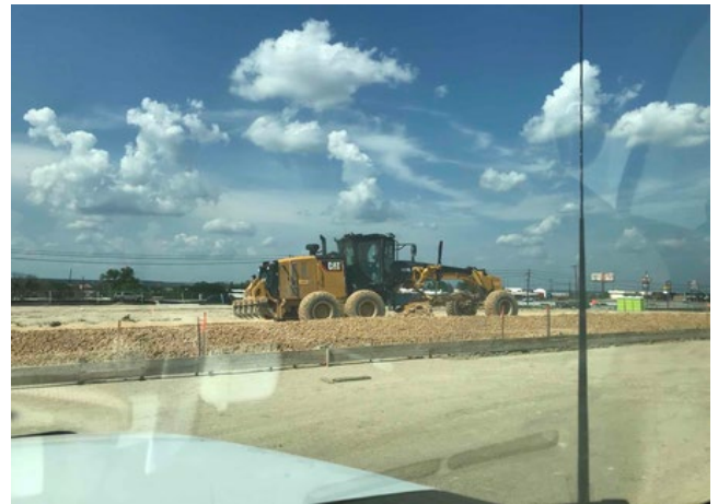
Exterior: Beginning to see road top in preparation of concrete
