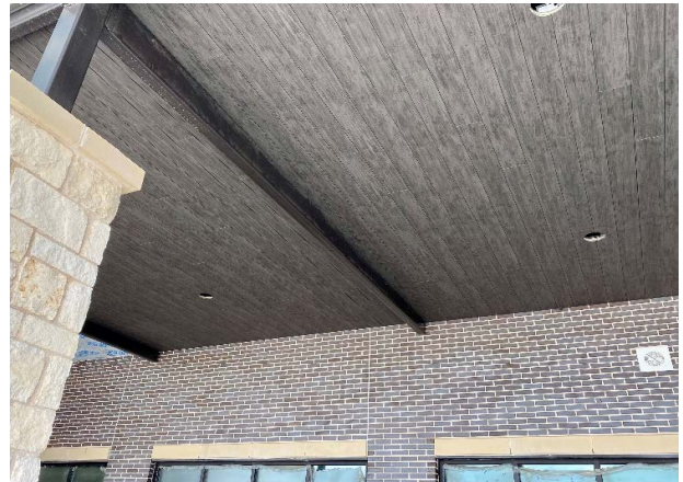
Exterior: Trespa ceiling install at front & rear canopy.
