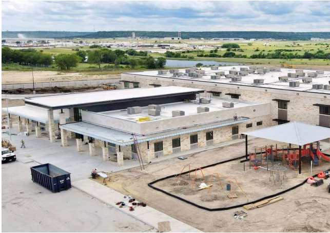
Exterior: Playground, top soil, irrigation and fencing are going in.
