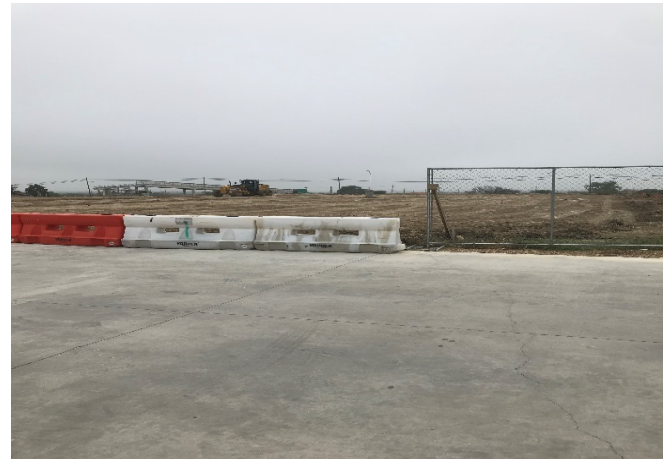
Exterior: Electric run for light poles and sleeves for irrigation.
