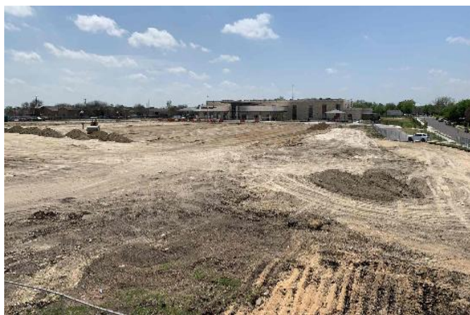
Exterior: Grading and fill.
