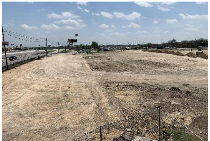
Exterior: Grading and fill.
