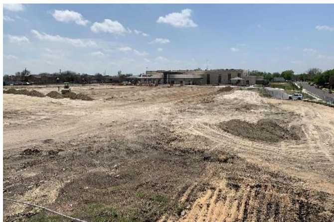
Exterior: Grading and fill.
