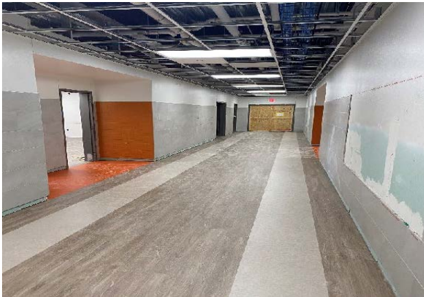
Interior: Hallway floor and wall tile install.
