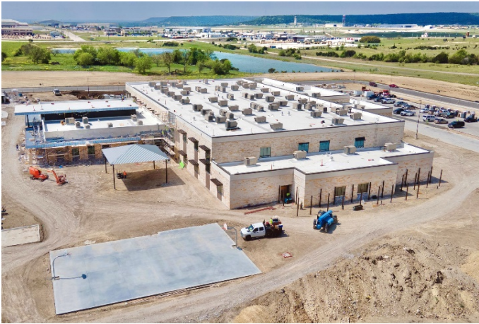
Exterior: Avadek canopies have begun, continuing sidewalks around property.
