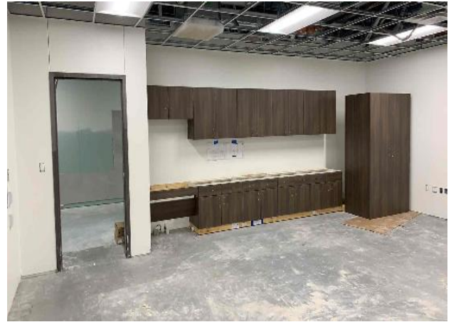
Interior: Casework has arrived and is being installed.
