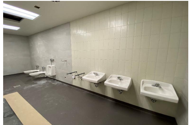
Interior: Restroom fixtures are being installed.
