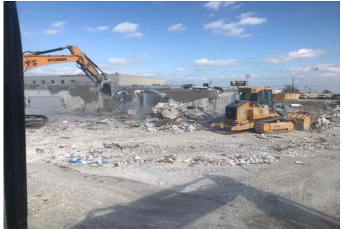
Exterior: Demolition of old building.
