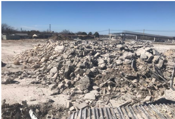
Exterior: Entire old building is demolished. Haul off has continued.
