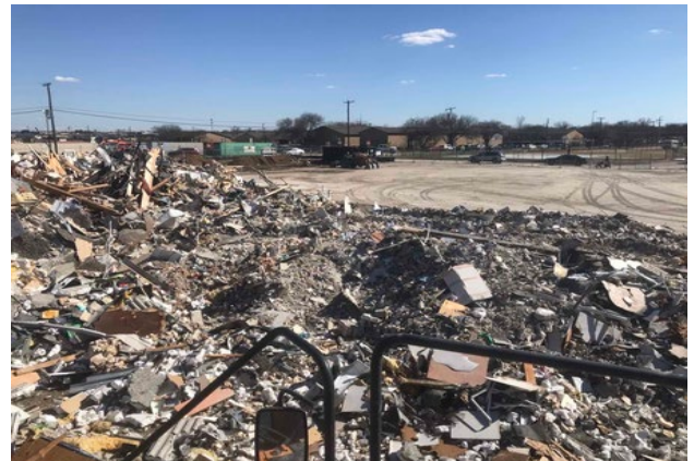
Exterior: Haul off of debris continues. .
