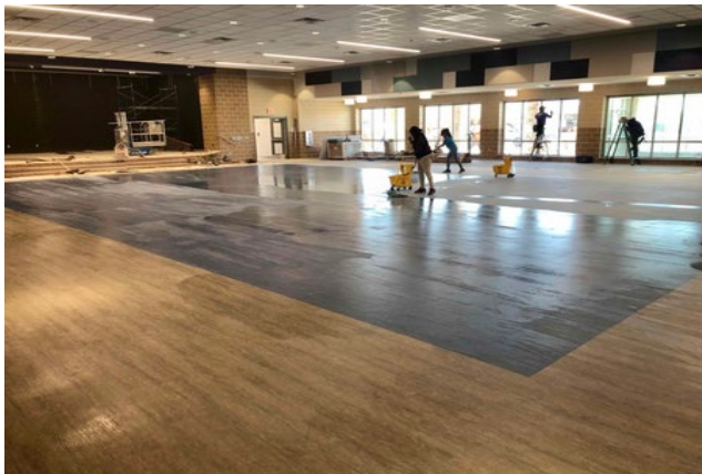
Interior: Cleaning and preparing for furniture delivery.
