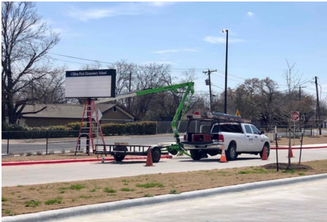
Exterior: Marquee installation.
