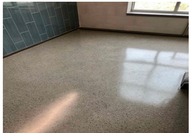
Interior: Terrazzo landings are poured and polished.
