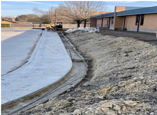
Exterior: Final retaining wall on East side.
