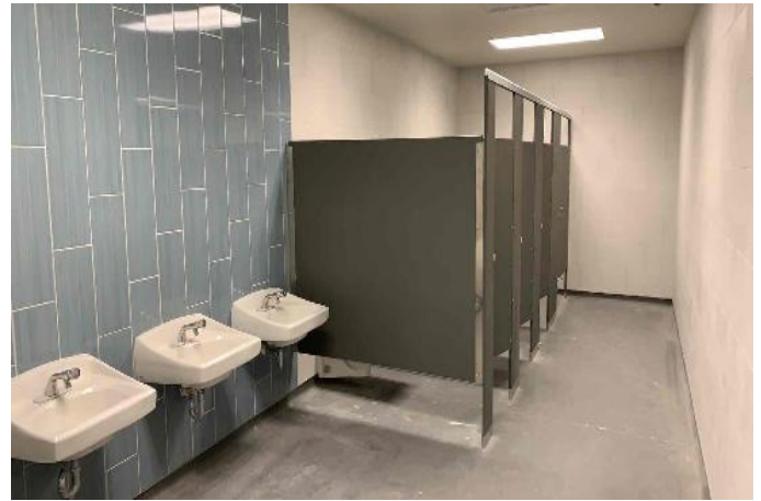
Interior: Bathroom partitions and accessories have begun install.
