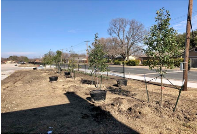
Exterior: Landscaping and trees have begun.
