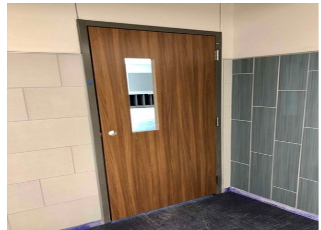
Interior: Classroom doors have begun installation
