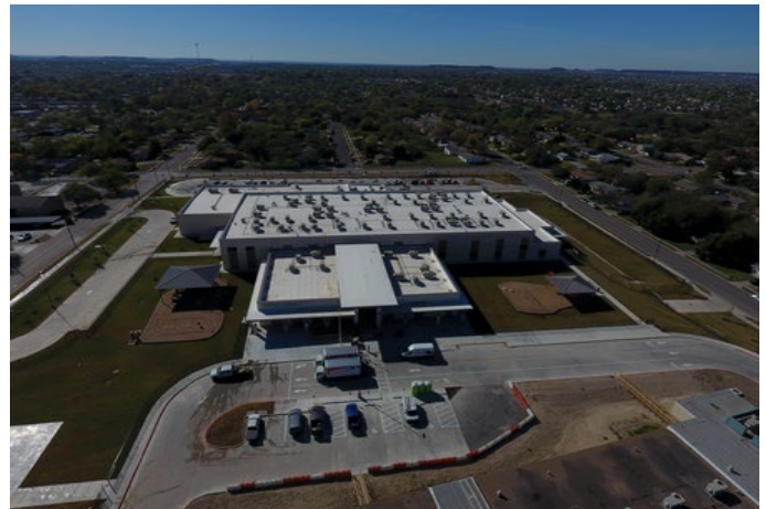
Exterior: Parking lot striping and signage
