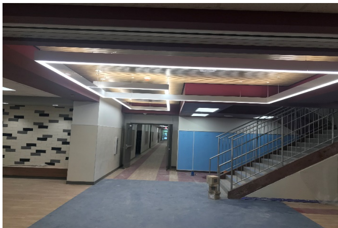
Interior: Final cleaning.
