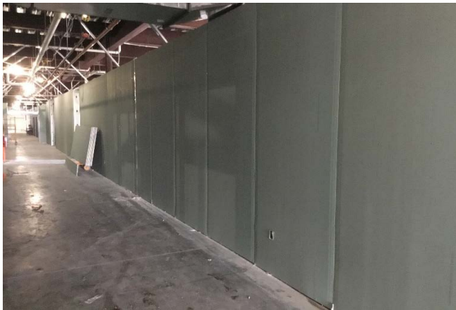
Interior: Area 3 interior walls sheetrock installed
