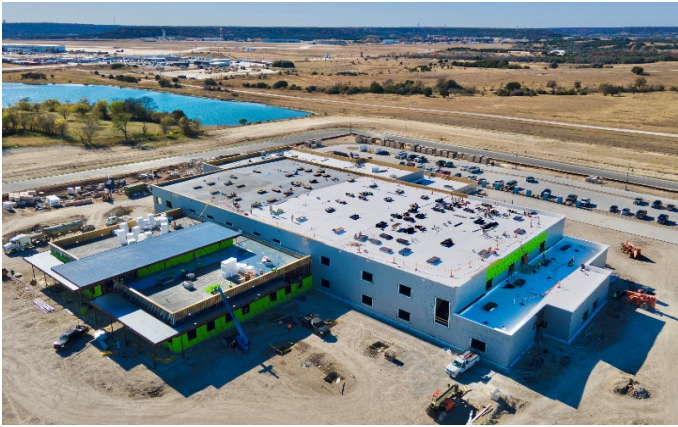
Exterior: Roofing in progress on Areas 5 & 6; starting on Area 1.
