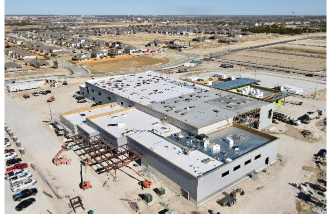
Exterior: Area 4 lightweight concrete to pour, rear canopy steel in progress.
