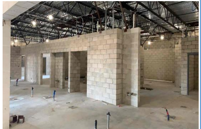
Interior: Area 4 Kitchen CMU walls completed.
