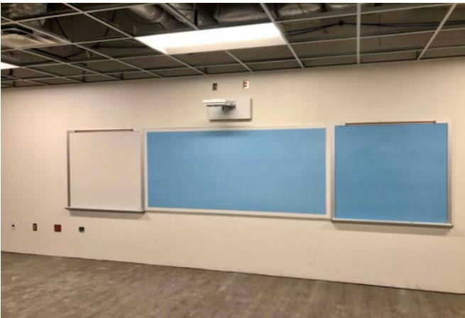
Interior: Classroom markerboards & projector mounts are being installed.
