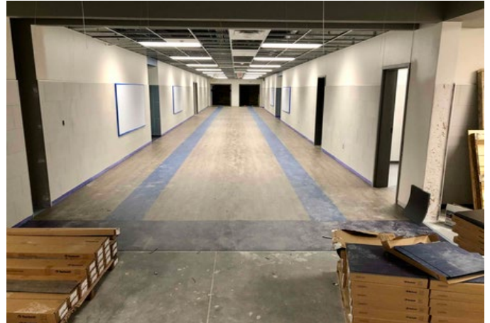
Interior: Classroom flooring downstairs finishing up and hallways in progress.
