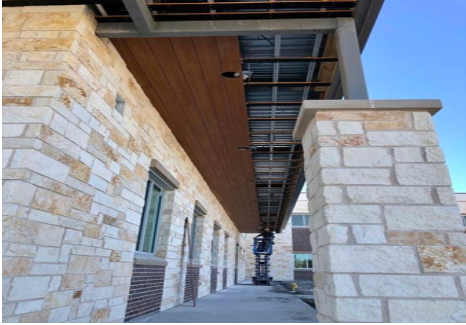
Exterior: Trespa ceiling install in front canopy.
