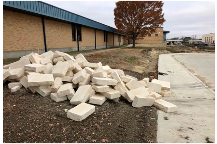
Exterior: Final retaining wall stone arrived for install.
