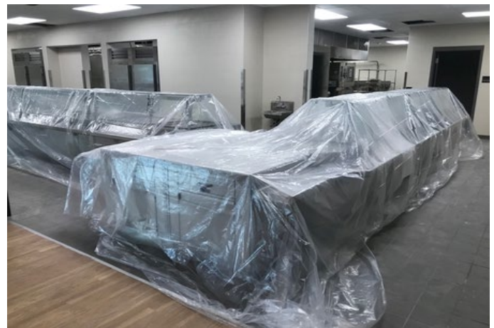
Interior: Kitchen serving line is installed and protected.
