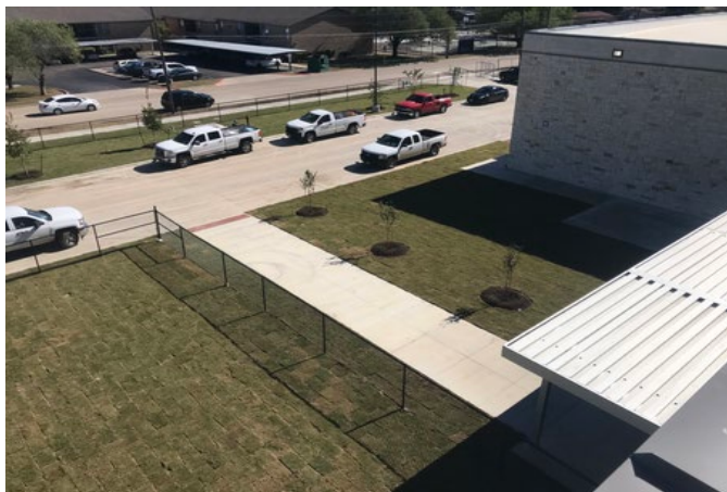
Exterior: All landscaping and sod has been installed.
