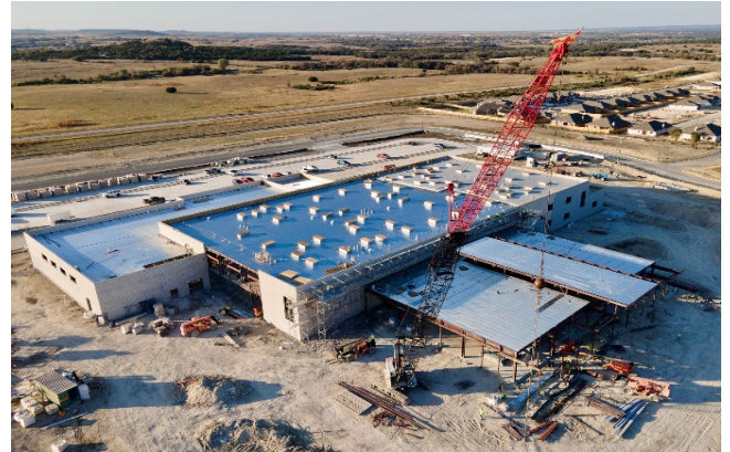
Exterior: Drone view; Area 1 roof decking and canopy steel.
