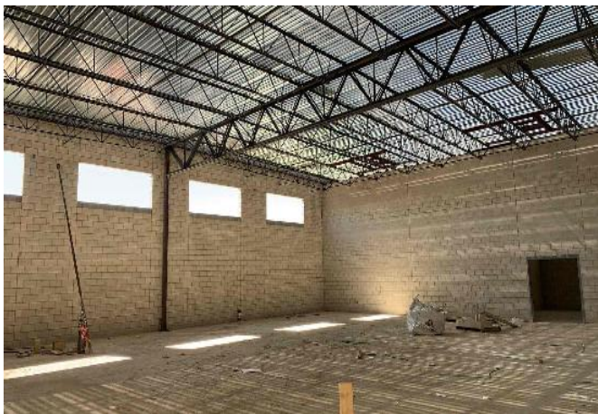
Interior: Area 4 CMU completed and roof decking installed.
