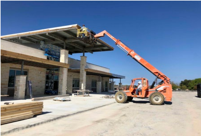
Exterior: Front canopy soffit installation preparing for finishes.
