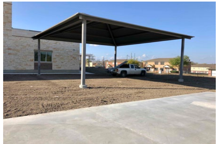
Exterior: Playground canopies are installed.
