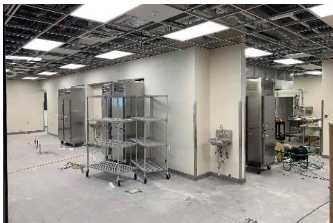
Interior: Kitchen equipment arrived and is being installed.
