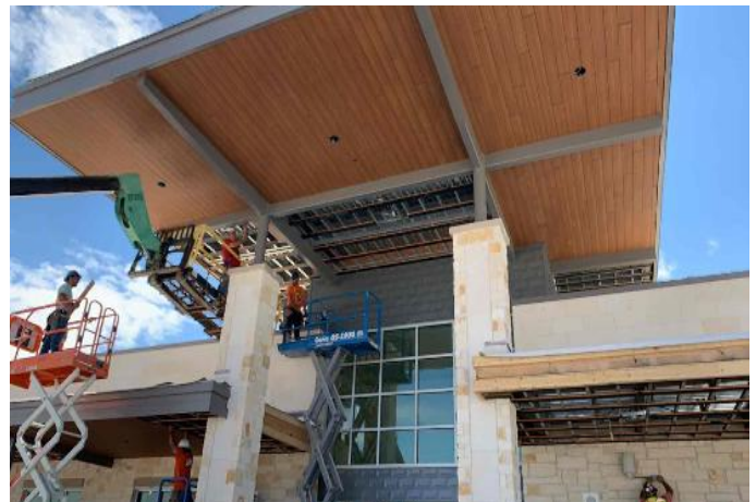
Exterior: Tresa wood installed in canopies.
