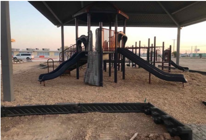
Exterior: Playgrounds are fully installed on both sides.
