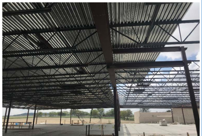
Interior: 2nd floor Area 5 & 6 roof decking install.
