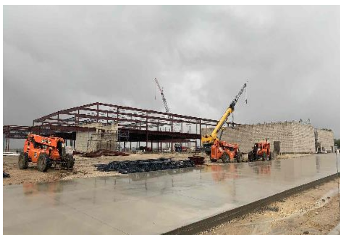
Area 2 & 5: Steel erection.
