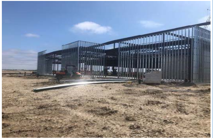
Area 3: Exterior Cold Form Metal Framing installed.
