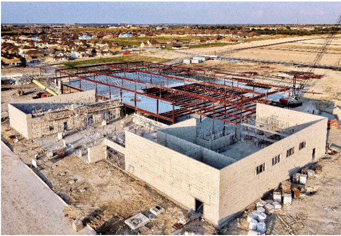
Exterior: Drone view from Southwest; PE and kitchen CMU install.
