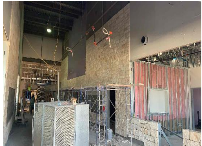
Section 1: Hallway stone wall tile outside of Administration.
