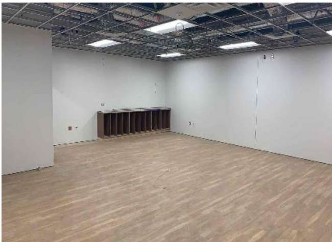
Section 2&3: Classroom floors, casework & ceiling grid.
