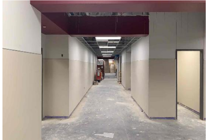
Section 2&3: First floor hallway wall tile finished.
