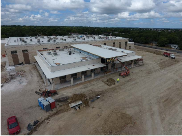
Site: Front aerial view, finishing column wraps.
