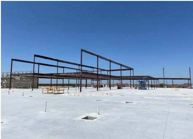
Section 3 & 6: Steel erection.
