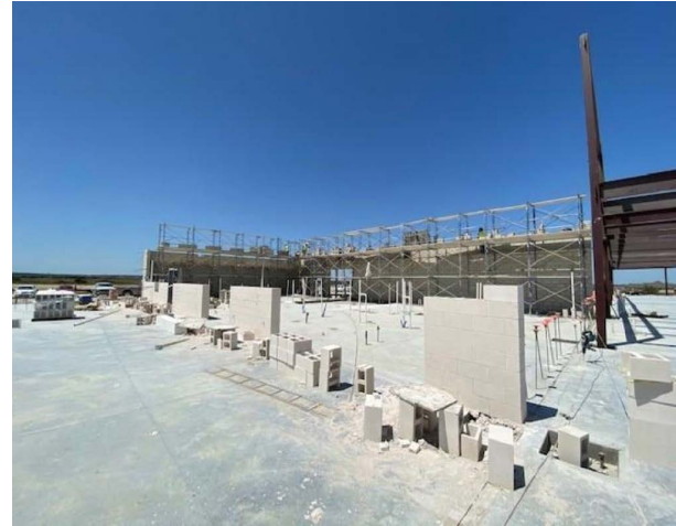
Section 4: Placing CMU.
