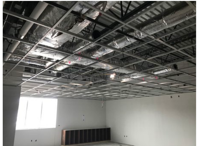
Section 2&3: Downstairs ceiling grids have begun install.
