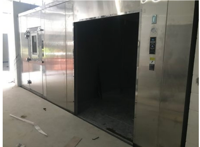
Section 4: Walk in freezer & refrigerator are being installed.
