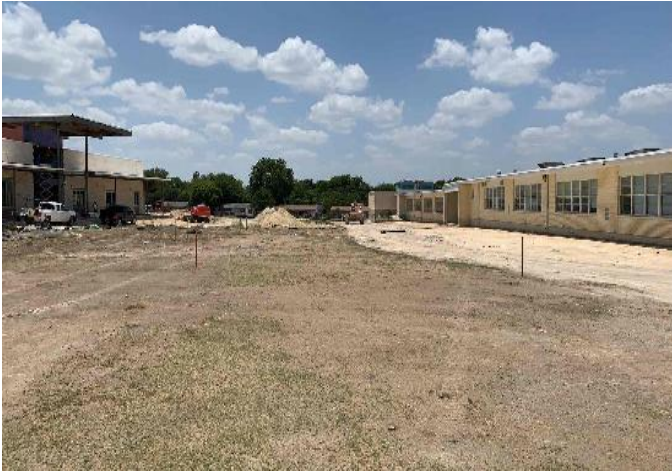
Site: Front grading for parking lot set to begin.
