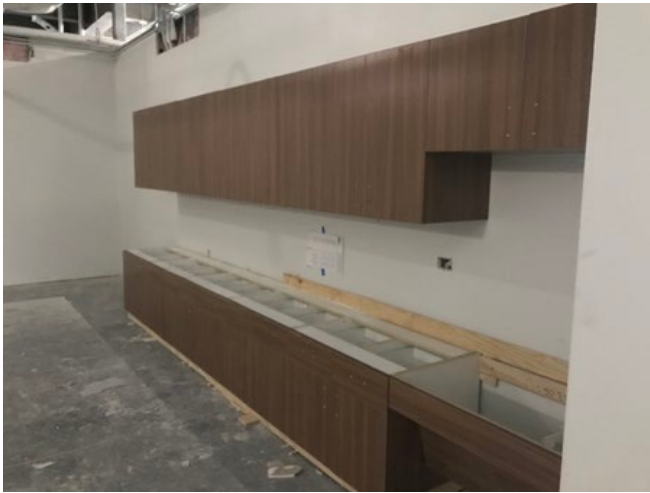
Section 2&3: Classroom casework has begun.
