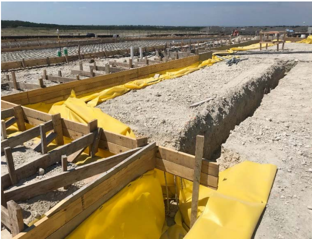
Site: Section 4 grade beams forming.
