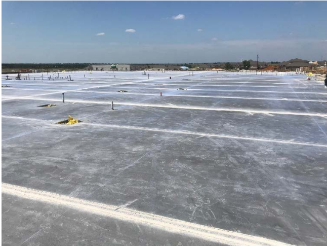
Section 3: Section 3 slab poured.
