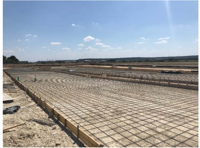
Site: West parking lot prep for concrete.
