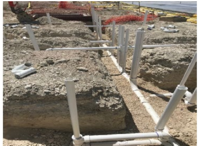
Section 2: Underground plumbing continues ahead of slab.
