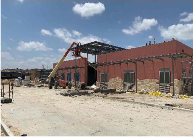
Building: Front entry canopy install.
