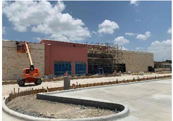
Building: Rear drive and masonry install.
