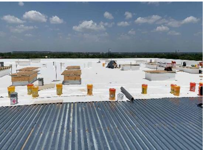
Section 4: Roof membrane install over main roof.
