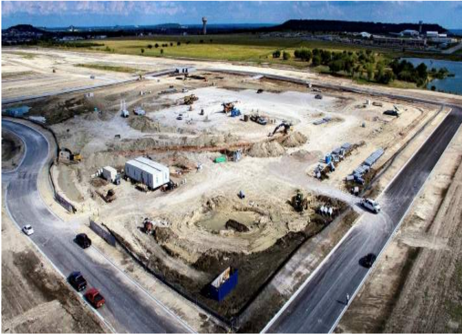
Site: Arial from Northeast.
