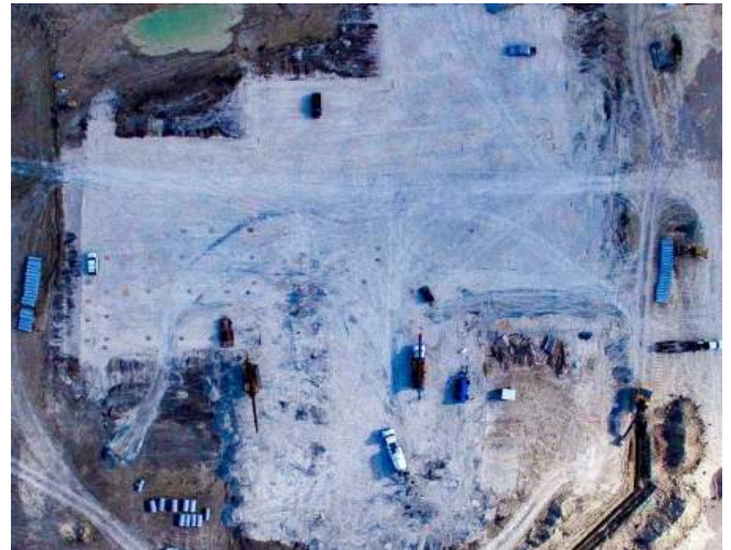
Site: Site overview pier drilling.
