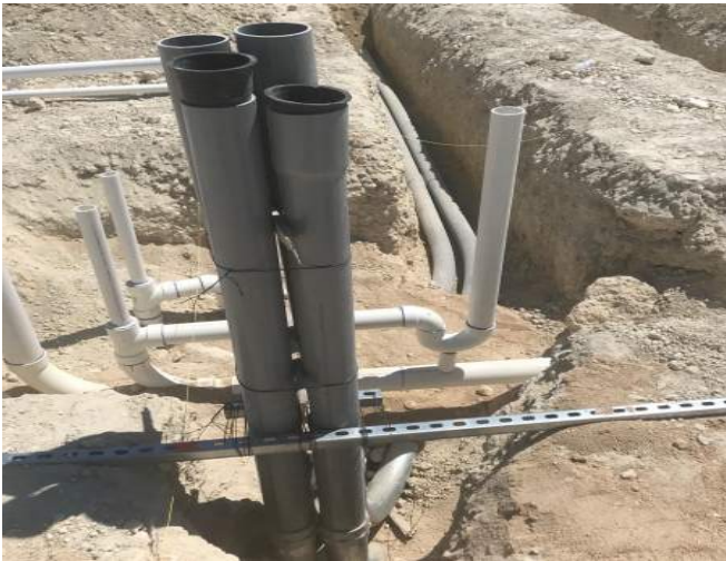
Site: Underground electrical and plumbing.
