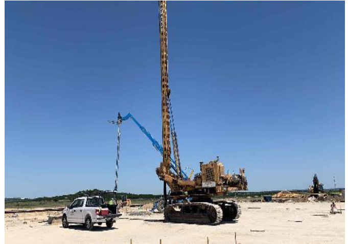
Site: Drilling Piers
