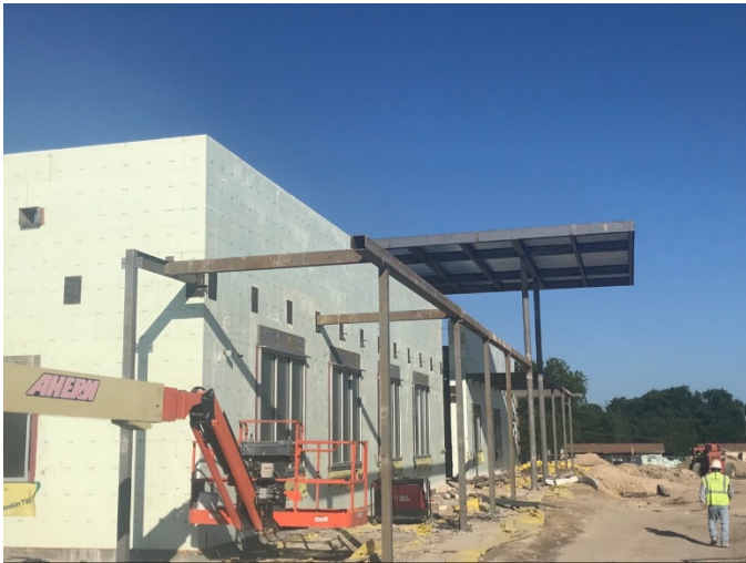
Section 1: Steel for front canopy being installed.
