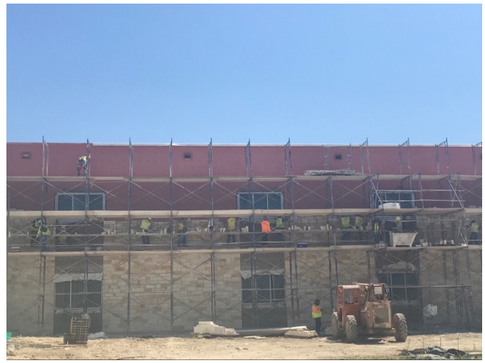
Section 2: Stone work is continuing around the building.
