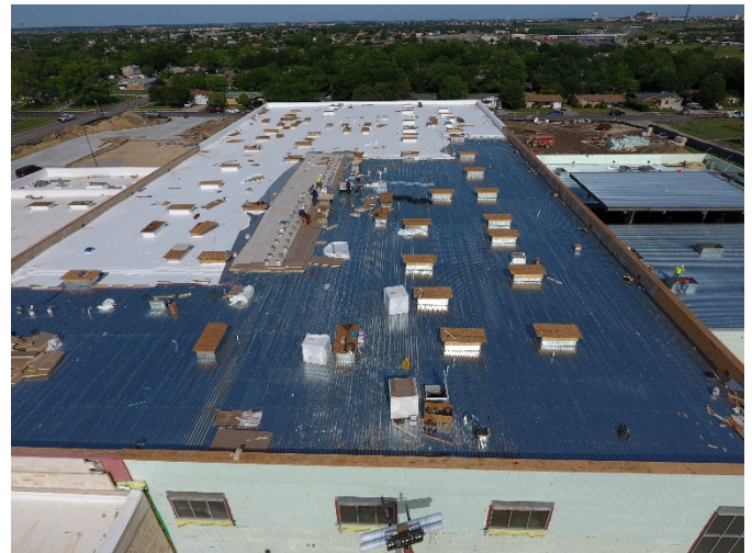
Section 5 & 6 Roof: Roofing in progress with rooftop units to follow
