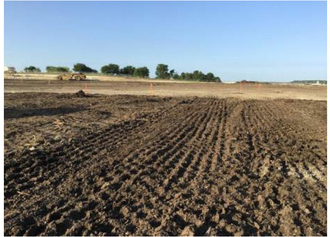
Site: Cutting site.
