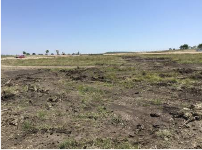
Site: Clearing and grubbing site.
