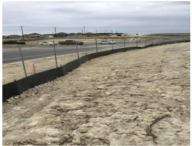
Site: Installed construction fence and silt fence.
