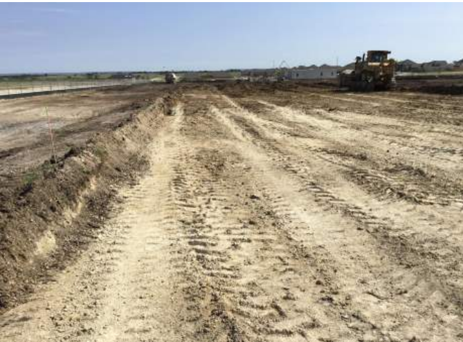
Site: Ext. Cutting temporary sediment ponds
