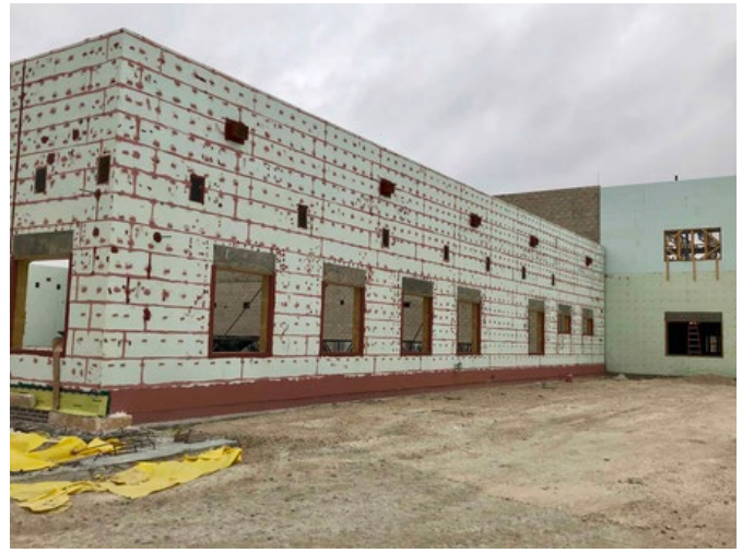
Sections 1: Waterproofing and sealing of walls
