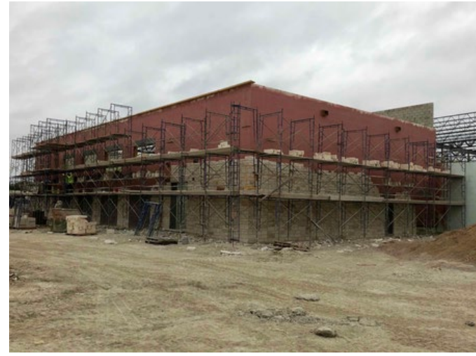
Section 2: Stonework in progress moving around the building.
