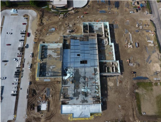
Building: Overview from the west.
