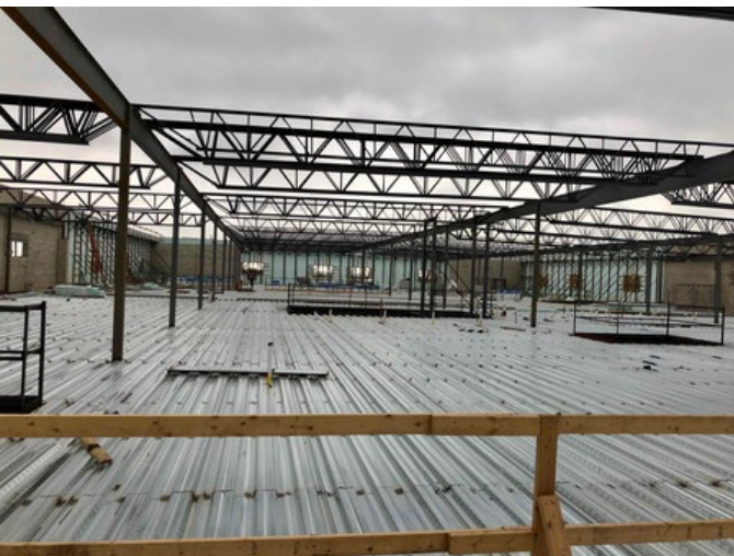
Section 5 & 6: Decking and preparing for 2 nd floor slab pour.
